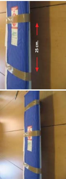
The heat blanket must have contact to the surface that shall be heated. In this case done with tape 25 cm between the tape fixation
